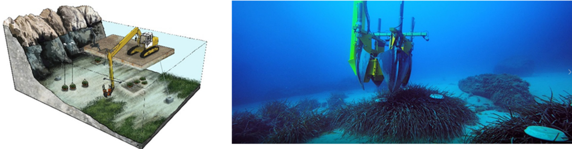
Figure 10. (Left) The excavator, on a pontoon anchored to the bottom. From Descamp et al. [236]. Courtesy of the author. (Right) A view of the clod transplanter in operation. Photo © Andromède océanologie. Courtesy of the author.
